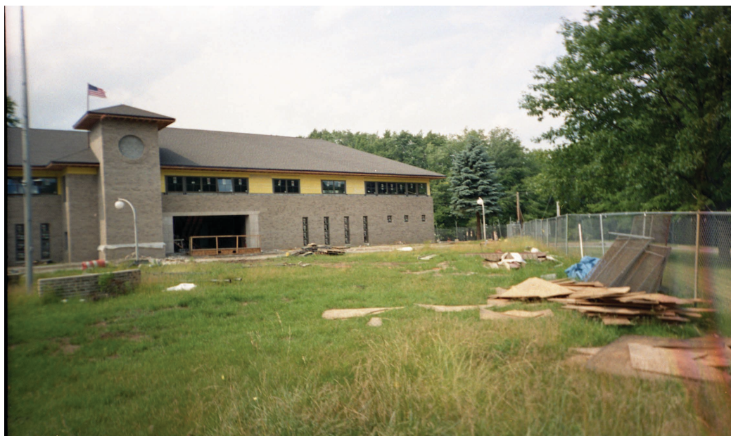
Figure 5 Municipal Building Under Construction Circa 2000. Note second arch added.
