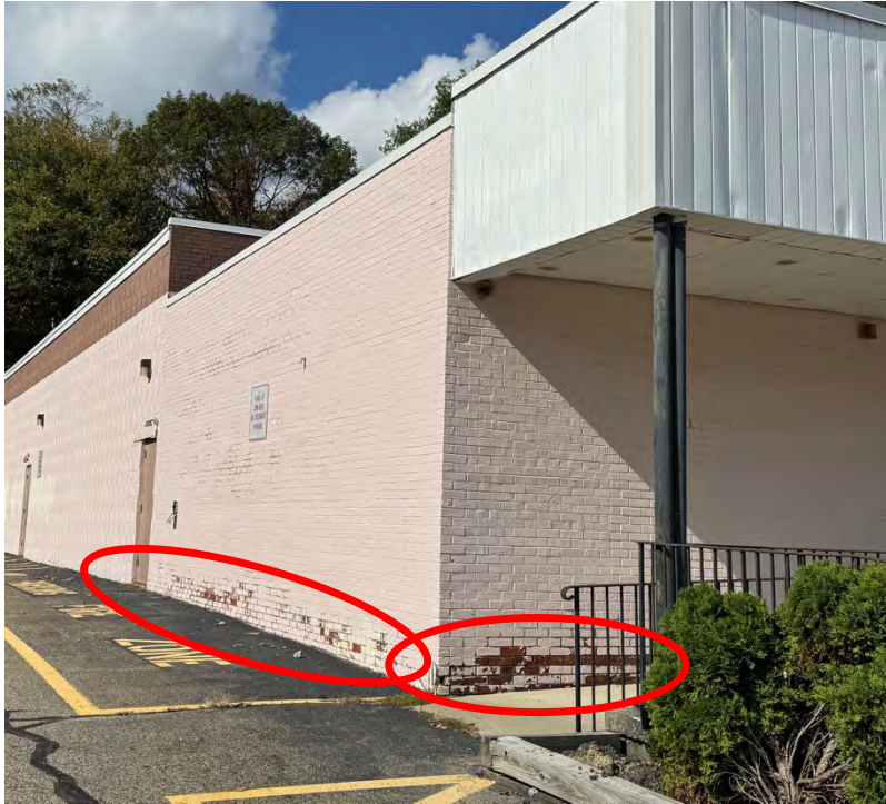
Above: Front and southern side of building with missing masonry and holes in the exterior wall.
