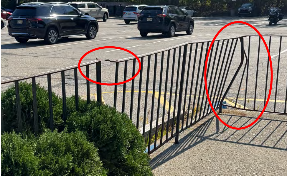
Above Front railing in need of replacement.
