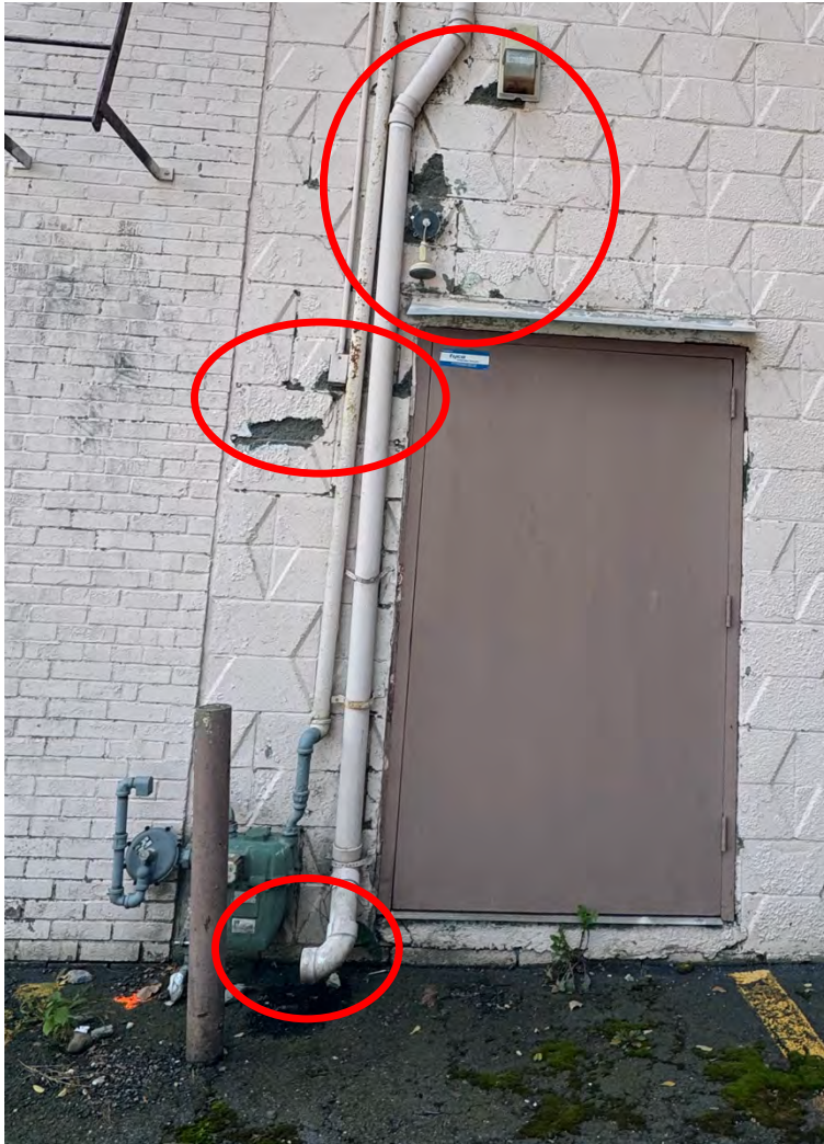
Left: Northern side of building with masonry loss and holes, as well as the building gutter which empties to parking lot without collection.
