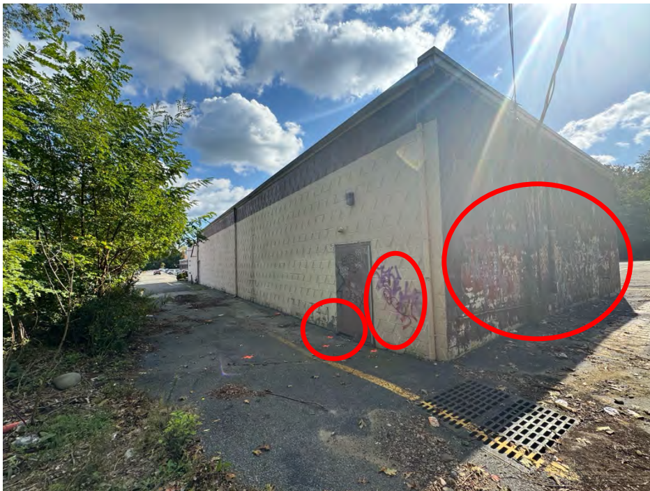
Above: Rear and northern side of building with extensive graffiti, missing masonry and deterioration of the exterior door.
