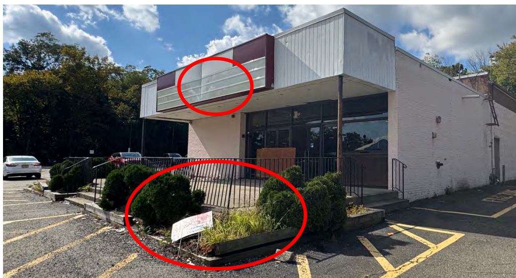
Left: Building front, facing south, with dents and a collapsed planting bed.
