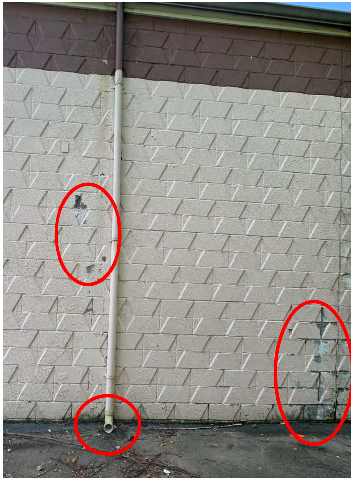
Above and left: Northern side of building with loss of masonry and holes, and deterioration of the exterior door, and a gutter which empties to the parking lot without collection.
