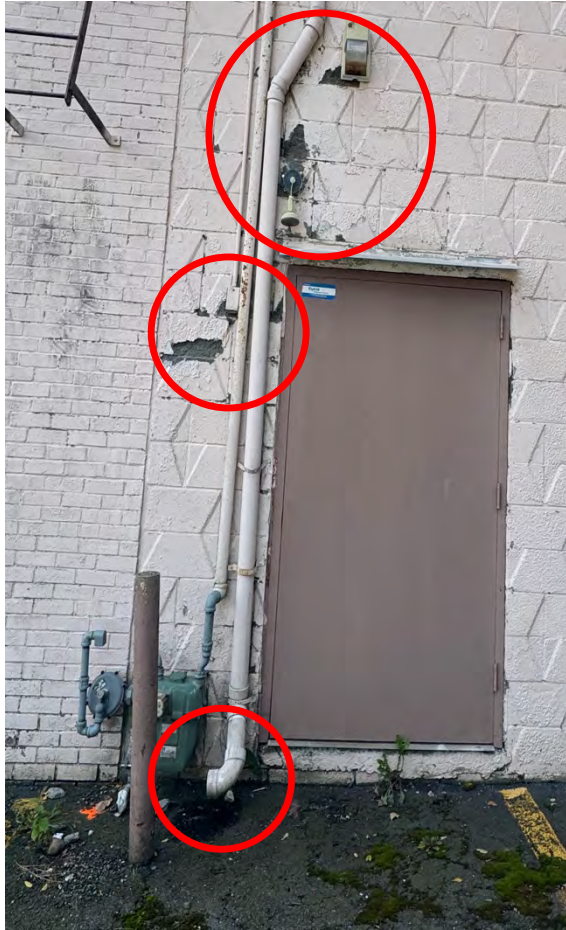
Left: Northern side of building with masonry loss and holes in the building exterior, as well as a gutter which empties to parking lot without collection.
