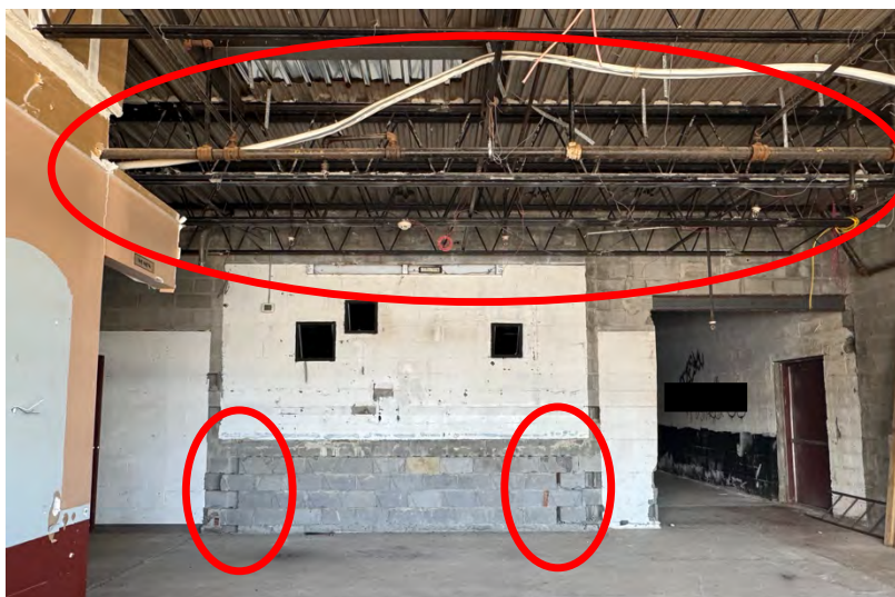
Above: Graffiti, exposed wires, missing masonry and graffiti (graphic graffiti has been redacted).
